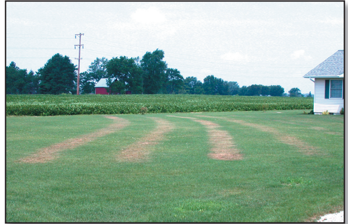
Figure 1. Brown turfgrass over soil absorption field trenches indicates an absorption field that is probably functioning as designed.
