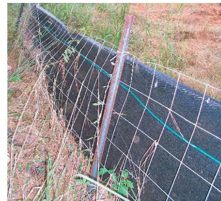
Use wire-reinforced silt fence and steel posts to reinforce sections downstream of large areas.
