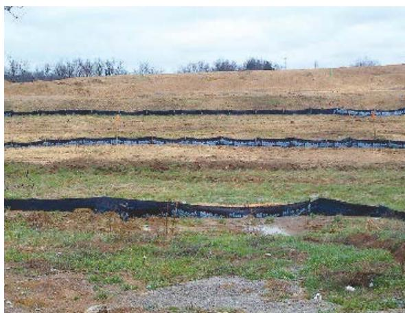
Use multiple sections of silt fence to interrupt long slopes.
