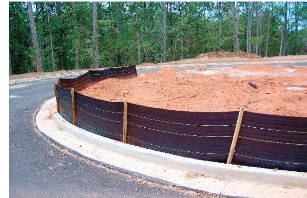
Silt fencing is commonly used to pond, settle, and filter sediment from sheet runoff. On slopes; set back from slope toe to allow for maintenance. Make sure fencing is trenched in properly and stakes are on the downhill side. Inspect frequently to detect and address bypasses, undercutting, and overtopping.
