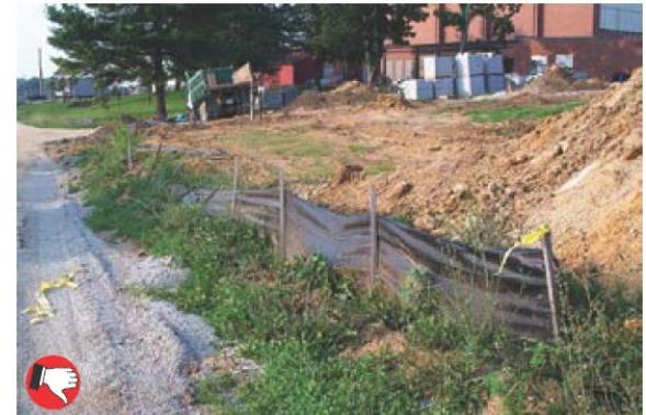
Inadequate maintenance of silt fence.
