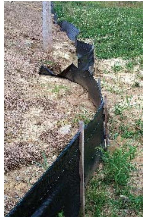
Silt fence functioning but in need of cleaning and replacement.
