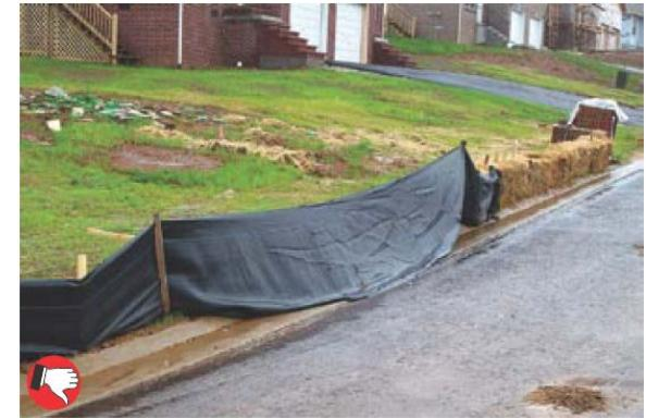
Improper trenching of silt fence.
