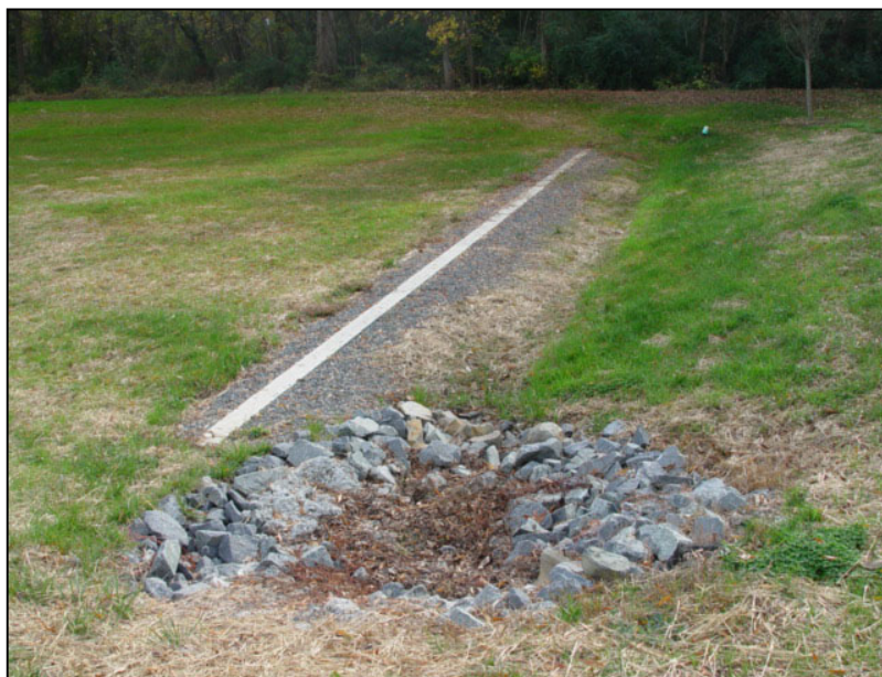
Figure 1 Level spreader, Charlotte, NC (NC State University)
