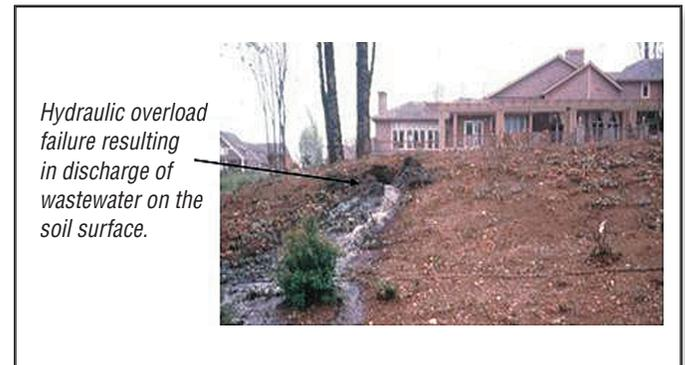
**Figure 2.** This photo shows an example of a septic system failing due to hydraulic overload. The soil absorption field could not accept the volume of water discharged from the home, resulting in septic tank effluent coming up to the ground surface.
