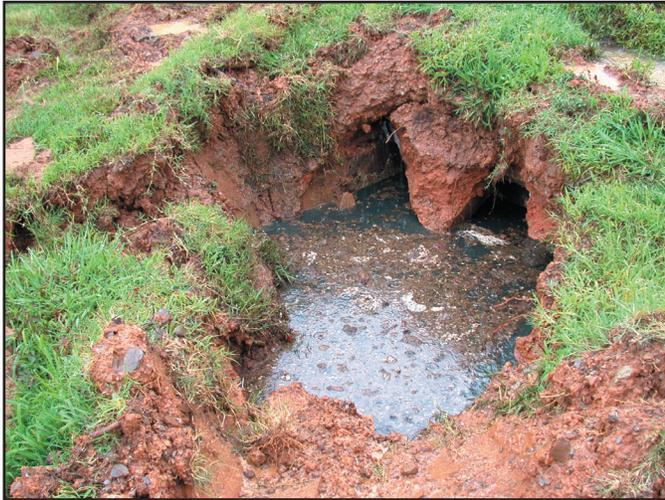
**Figure 4.** This photograph shows a concrete septic tank lid that has collapsed under a truck's weight. Repair costs were more than \$1,000.
