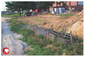
Inadequate maintenance of silt fence.
