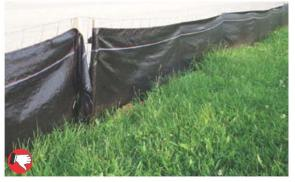
Two sections of silt fence not properly connected. Sections should be overlapped and wrapped together.
