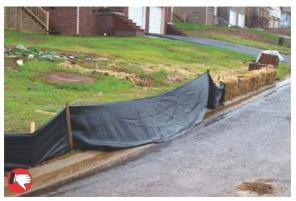
Improper trenching of silt fence.
