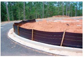
Silt fencing is commonly used to pond, settle, and filter sediment from sheet runoff. On slopes; set back from slope toe to allow for maintenance. Make sure fencing is trenched in properly and stakes are on the downhill side. Inspect frequently to detect and address bypasses, undercutting, and overtopping.
