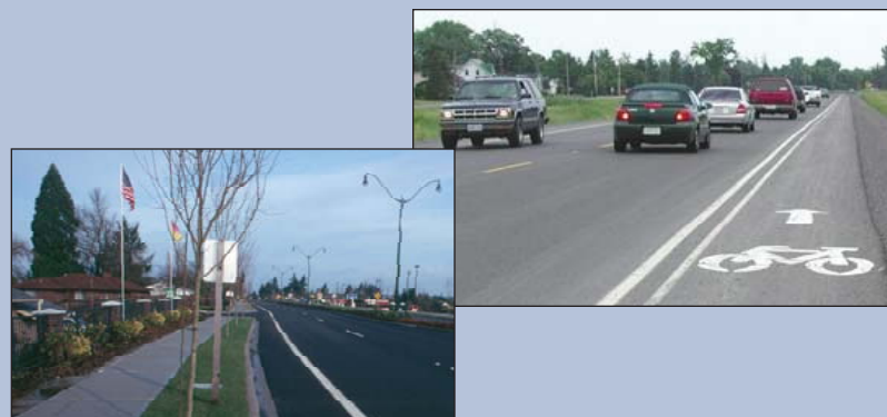
Complete streets: A bicycle lane on a rural road (above right) and room for pedestrians and bicycles along a commercial corridor (above left).
