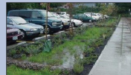
Innovative bioswale stormwater treatment along minor roads and parking lots.
