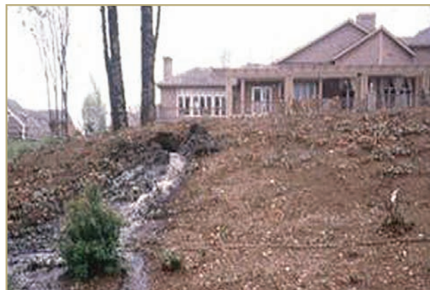
Figure 3. Septic system failure, which can be caused if the biomat at the soil-trench interface becomes too thick for wastewater to flow through, often results in septic tank effluent surfacing on the lawn.
