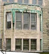
**Cornice** - is the uppermost section of moldings along the top of a wall or just below a roof.
