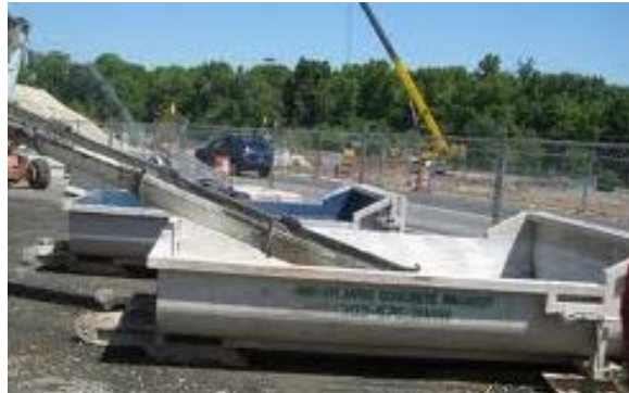
Self-contained sturdy containment systems that are delivered to a site and located at strategic locations for concrete washout.
