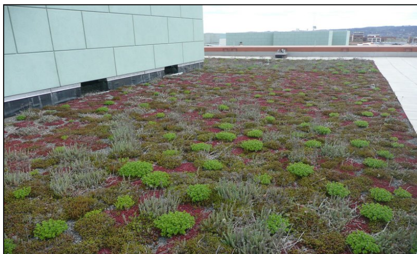
Figure 1 Vegetated Roof, Washington, DC (USEPA, picasaweb)
