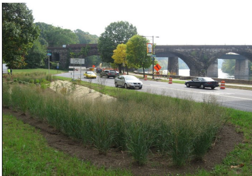
Figure 1 Vegetated Swale, Philadelphia, PA (USEPA, picasaweb)
