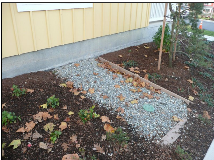
Figure 1 Infiltration Bed, Seattle, WA (USEPA, picasaweb)
